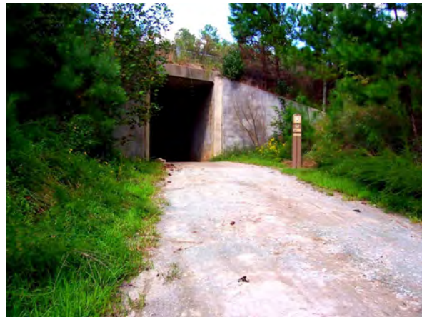
Tunnel under Highway 64
