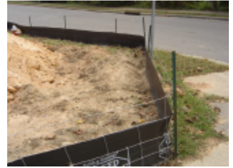
Shown above is an example of a steel-post, wire-back silt fence. This is the only silt fence accepted in the field by the Wake County Erosion Control Ordinance.
