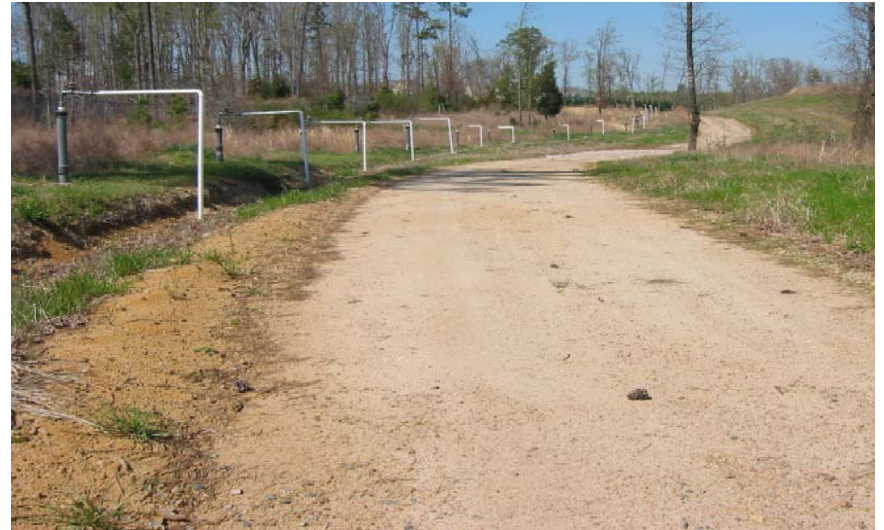
North Wake Gas Remediation Project
