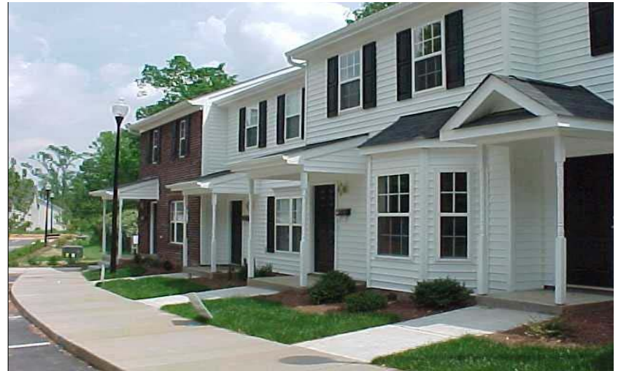
Callan Park at Waldo, Cary, 3 of 21 units in Townhouse Project
