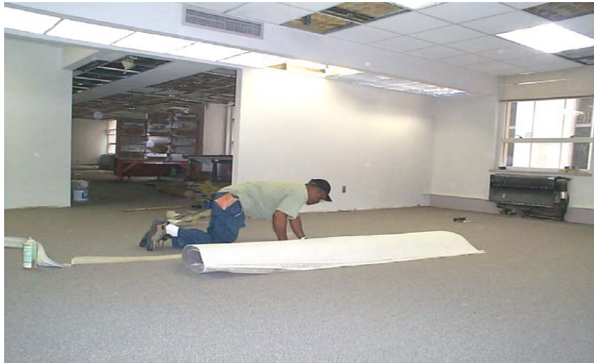
County Office Building 7th Floor Renovations
