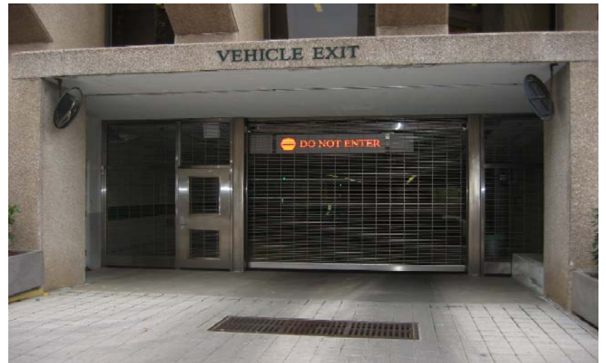
Courthouse Parking Gate Replacement
