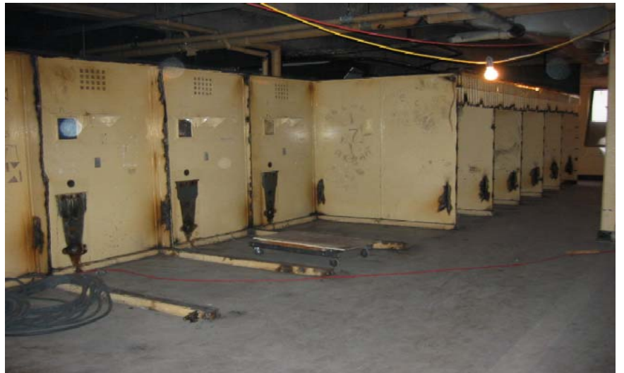
5th Floor Courthouse Renovation
