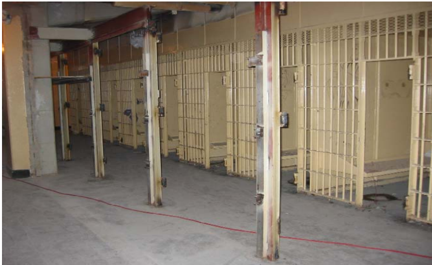
5th Floor Courthouse Renovation
