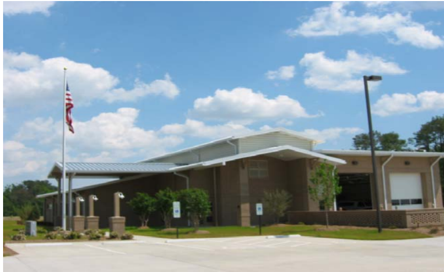
Willow Spring Fire Station
