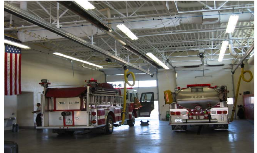
Willow Spring Fire Station Bays
