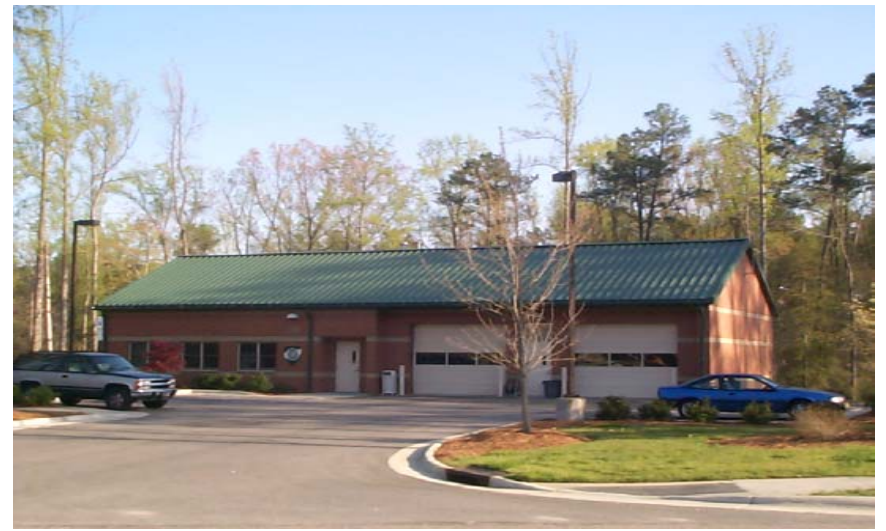
EMS Station at Kidd Road
