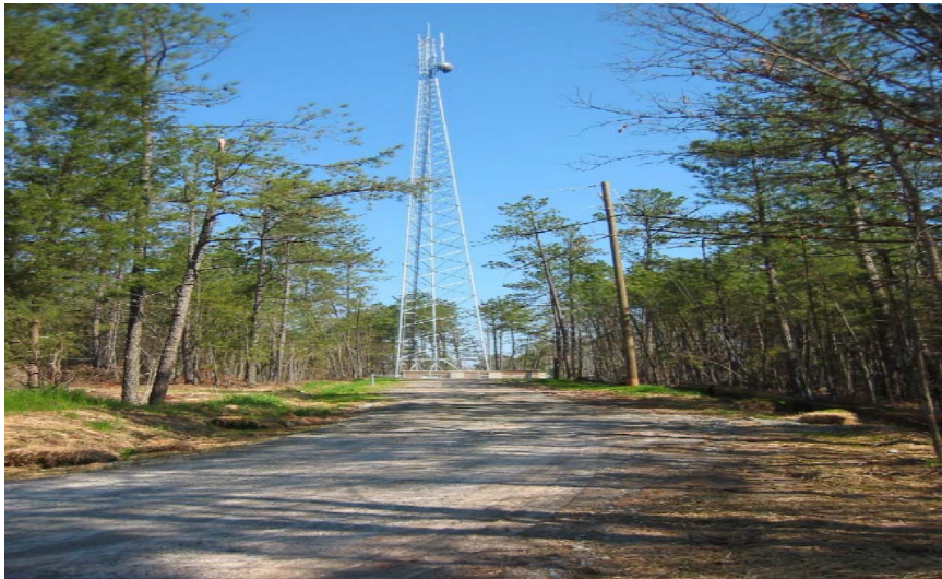
Radio Communications Tower, Research Triangle Park
