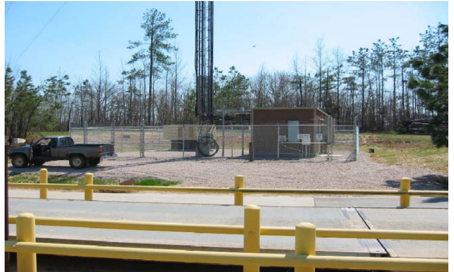
Radio Communications Tower, Northern Wake County
