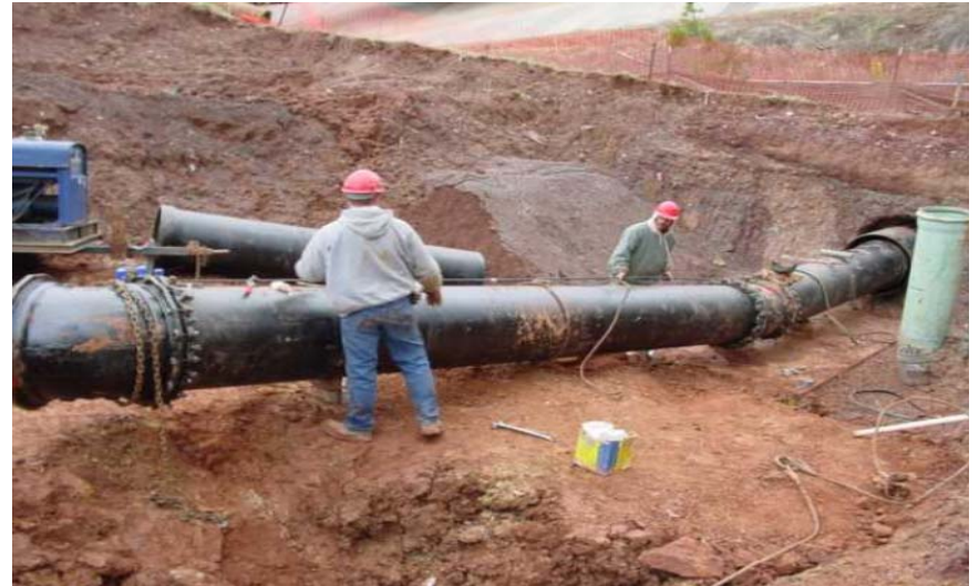
Water Sewer Line
