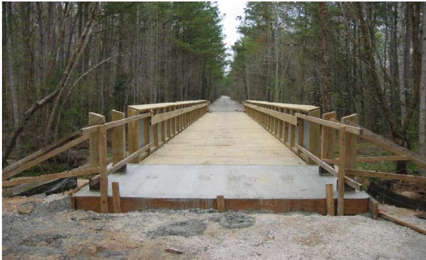
Reedy Branch Bridge, American Tobacco Trail
