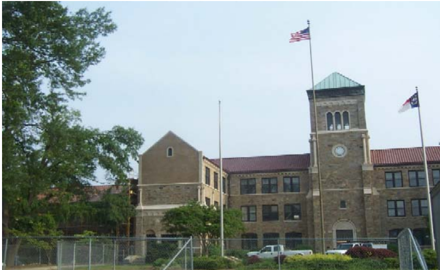
Broughton High School (Renovation Project)
