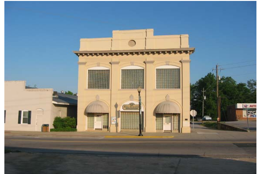
Former Apex Town Hall
