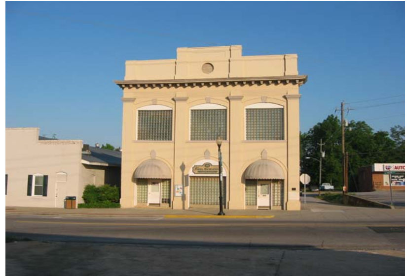
Former Apex Town Hall
