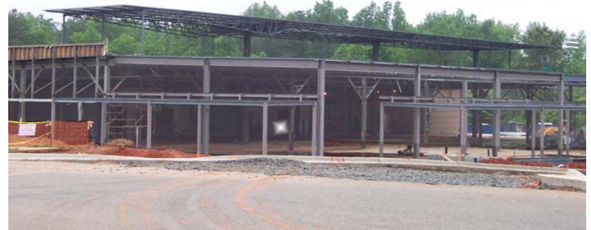
North Regional Library Construction Site
