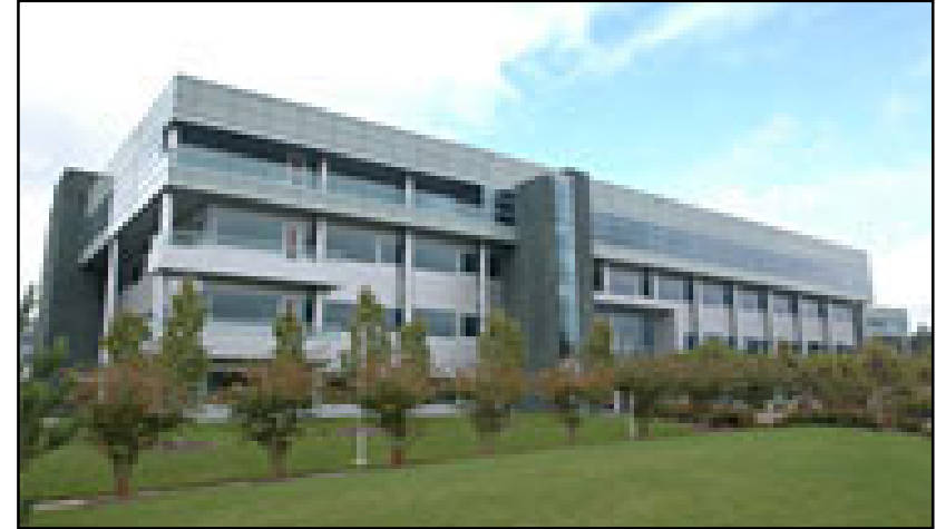
Credit Suisse First Boston Facilities in RTP South
