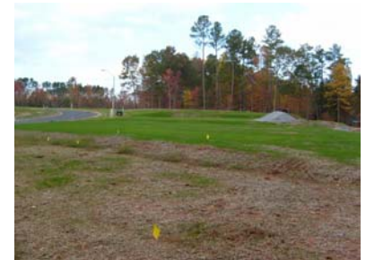
Bermuda grass seed, straw and asphalt tac
