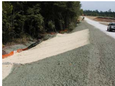
Lovegrass hydroseed and matted pipe crossing
