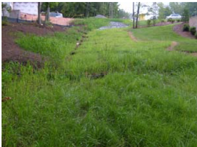
Netted wood mulch with biodegradable sock check dams
